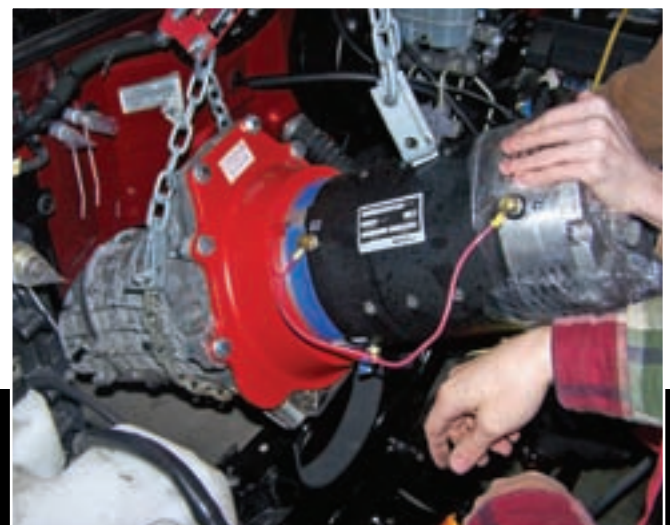
Installing the new electric motor and transmission, with room to spare.
